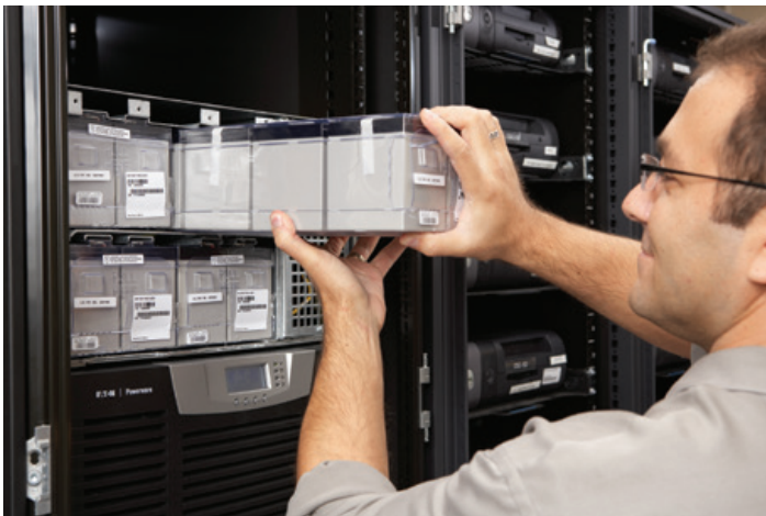
IT staff can easily replace battery modules.
