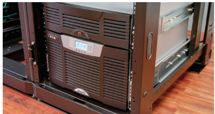
12 kW BladeUPS with extended battery module (EBM)
