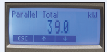
Display full system output from any UPS
